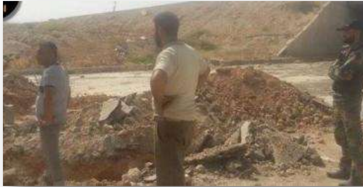
Fixing the water network in Al Nairab camp
