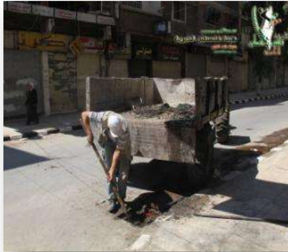
Cleaning the wastewater network in Yarmouk camp
