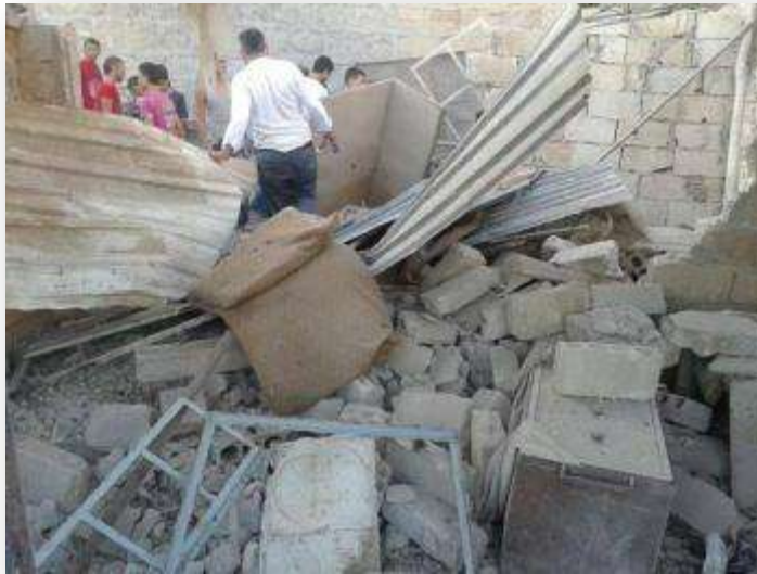
The damaged house in Alnairab camp
